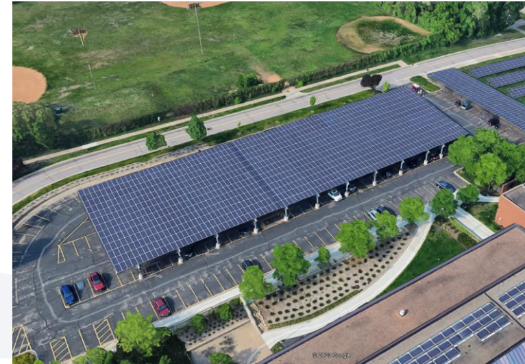
Parking Lot Carport PV Example
